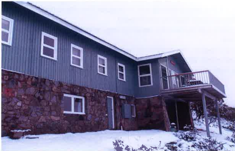
Photo 3.1 Shows existing building colours and materials to be matched
