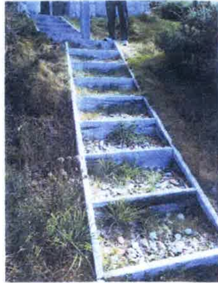
Stairs to front porch
