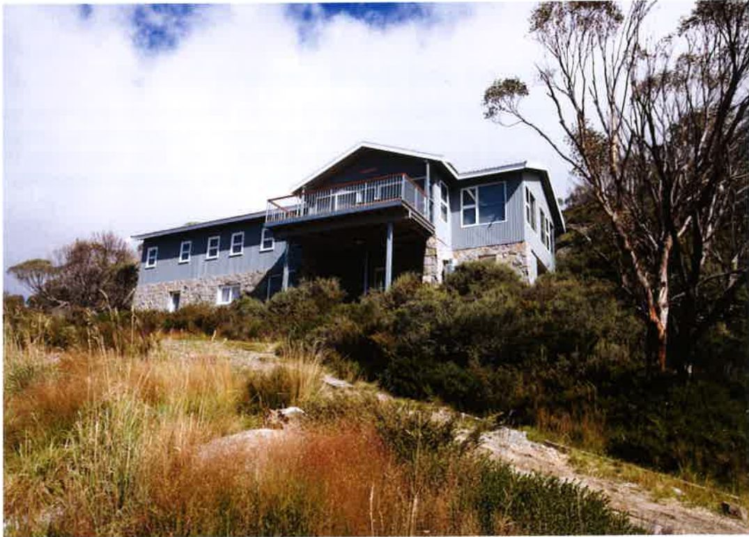
Photo 4.2 The existing visual nature of the Lampada Ski Lodge can be partly seen in the photo above.
