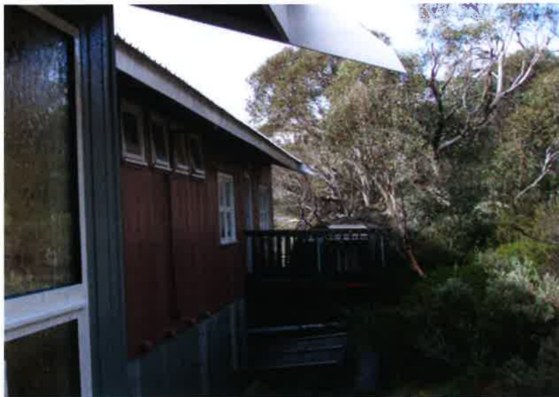
Photo 1.3 Section of the site in which the Broad-toothed Rat passage, scat and evidence of feeding was found with respect to proposed development area.
